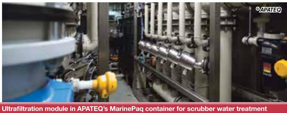
Ultrafiltration module in APATEQ's MarinePaq container for scrubber water treatment
